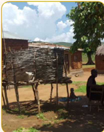
Traditional storage structures for maize in Mbeya and Ileje district. Referred to as 'vehenge'.
