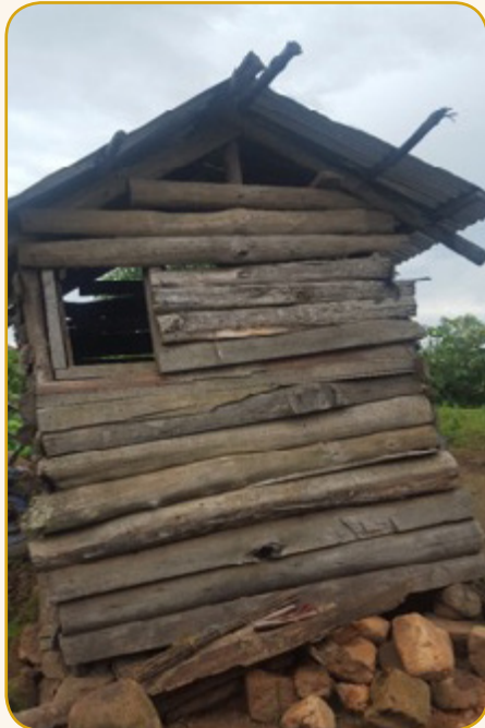
Traditional storage structures for maize in Mbeya and Ileje district. Referred to as 'vehenge'.
