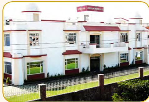
Arvind Chemi Synthetics facility in India.
