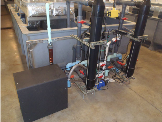
FIGURE 2. Photograph showing the 290-W W70D pump that comprises part of each RAS. Each system has one such pump and obtains water from two sumps. Water is diverted into the chilling unit and UV sterilizer before being distributed to the four linear tanks.
