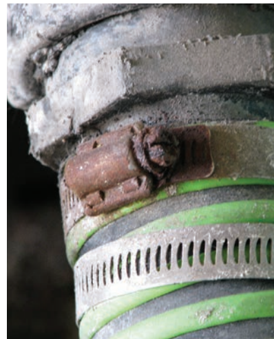
(Above) This disassembled worm gear clamp shows the interaction of the screw and the metal band. (Left) This rusted clamp needs to be replaced immediately.
