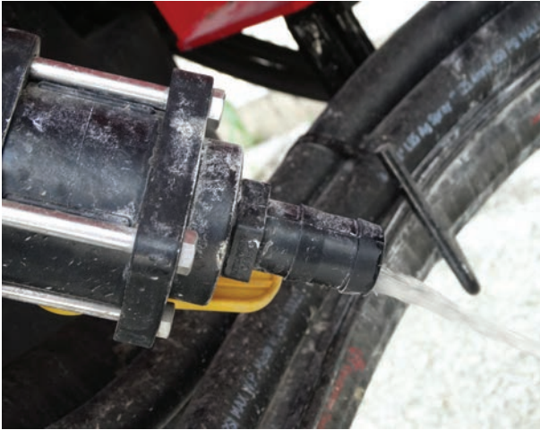
Opening all valves allows more water to be removed.
