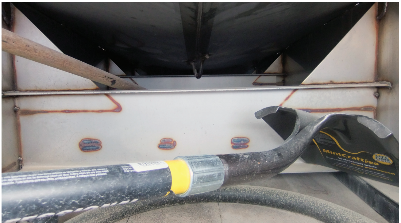
This picture shows the inside of the railing (sills). Notice the stainless steel cross members.
