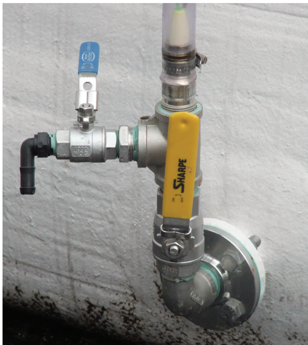
State regulations may require commercial agricultural dealers to provide regulators with a fertilizer sample to analyze and verify the product they are selling. This tank (left) has a small tap off the sight gauge, which provides an easy port to withdraw samples.
