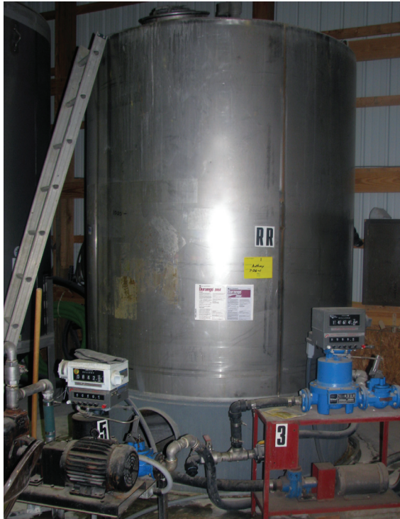
When placing a pesticide tank indoors, consider venting the fumes that come from the product to the outside of the building.
