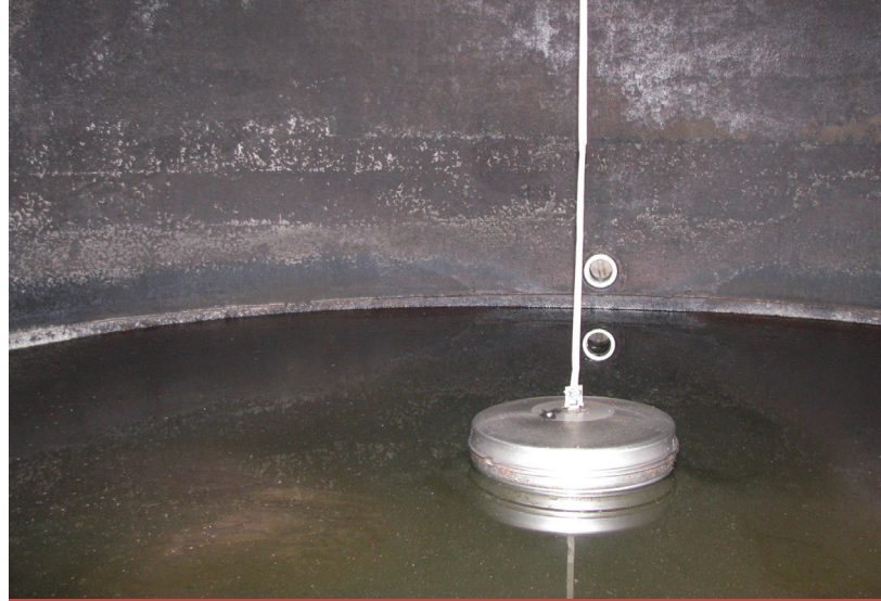
An internal sight gauge (above) normally is less vulnerable, but requires more maintenance. It is a good idea to consult the manufacturer so the style of measuring device you choose accurately measures the tank's contents.
