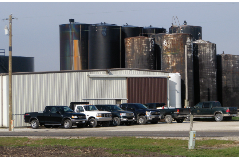
Used tanks can be a good investment as long as you know the condition of the tanks inside and out.
