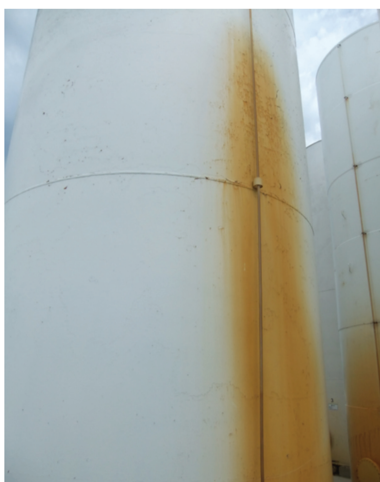
This tank looks like it developed a problem from a leaking line. General corrosion (such as rust) is mainly a cosmetic issue. A tank failure caused by general corrosion is a slow process.
