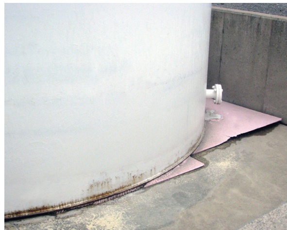
The bottom of this tank is showing signs of corrosion (left). Keep water away from the tank to help reduce corrosion next to the tank (middle and right).
