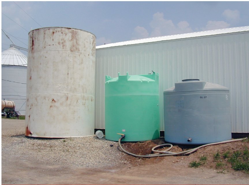
Every tank needs to sit on a solid foundation.
