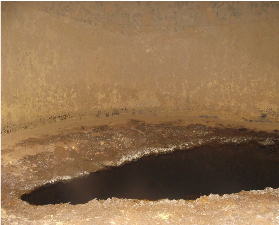
This tank was cleaned six years ago. Materials that are not agitated will salt out, and the residue tends to accumulate around the perimeter of the tank.
