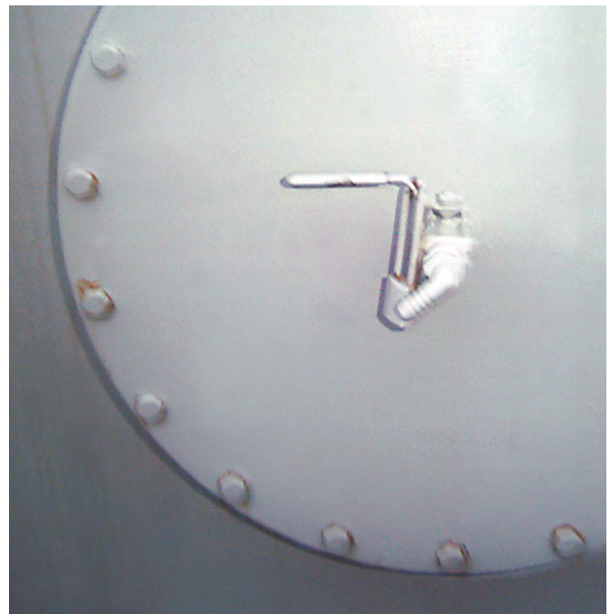
State regulations may require commercial agricultural dealers to provide regulators with a fertilizer sample to analyze and verify the product they are selling. This tank (left) has a small tap off the sight gauge, which provides an easy port to withdraw samples.
