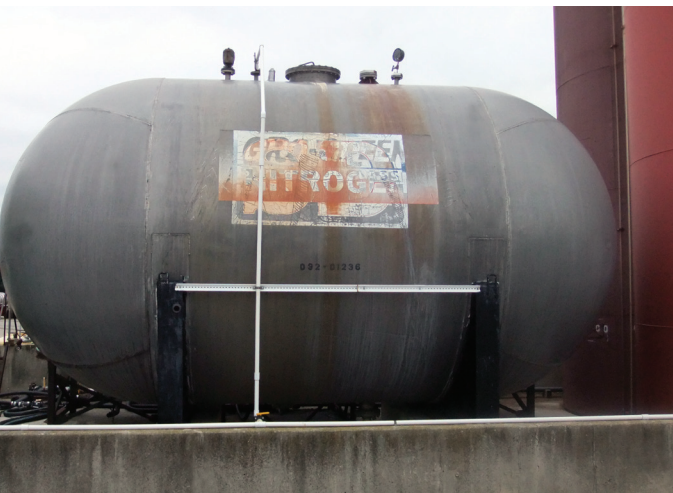
Based on the number of old decals, this tank that was built in 1964 and has been through many owners. The National Board of Boiler and Pressure Vessel Inspectors (National Board) identification number indicates the tank was built as a pressurized vessel. The concern is whether or not this is an aluminum tank. For a fee, the National Board can provide you with a tank specification sheet as long as the manufacturer's name and the board number are available. Call the National Board at 614 888 8320.
