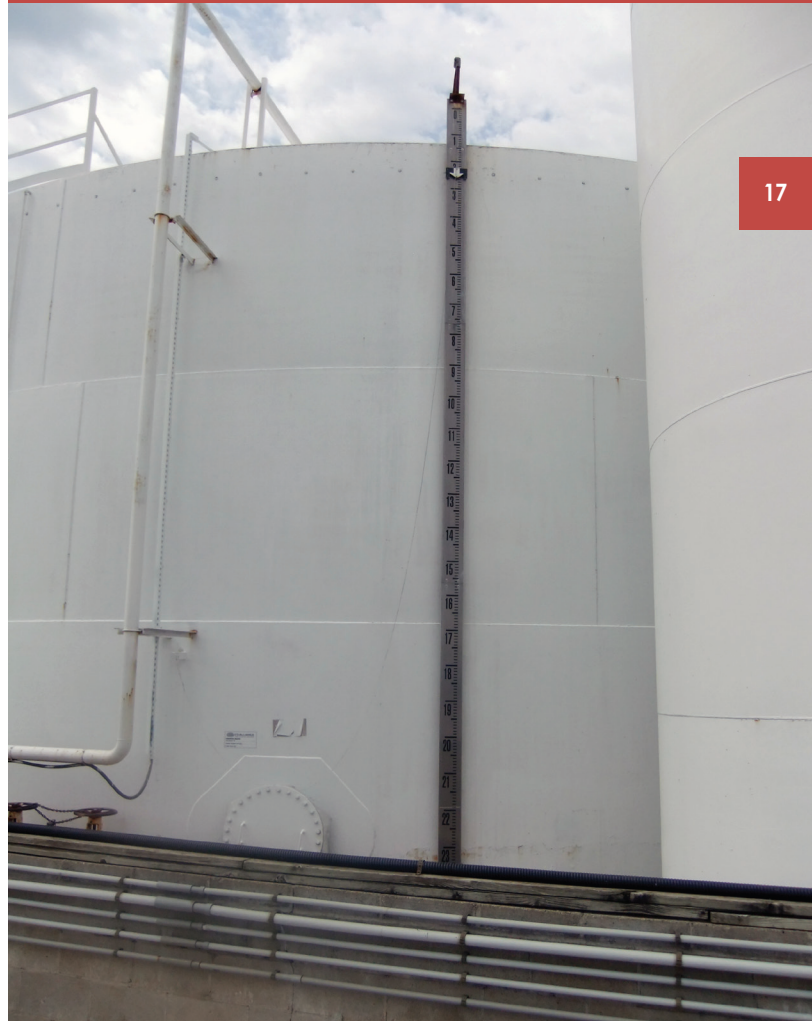
An internal sight gauge (above) normally is less vulnerable, but requires more maintenance. It is a good idea to consult the manufacturer so the style of measuring device you choose accurately measures the tank's contents.
