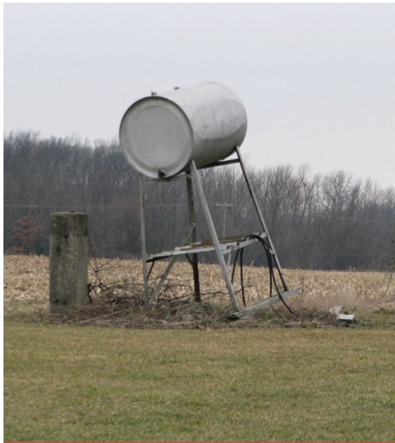
An unstable base will shorten the life of any tank.
