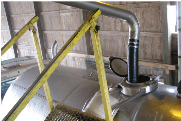
Keeping the fill port open while you fill the tank allows enough air to escape and prevent a seam or weld failure.
