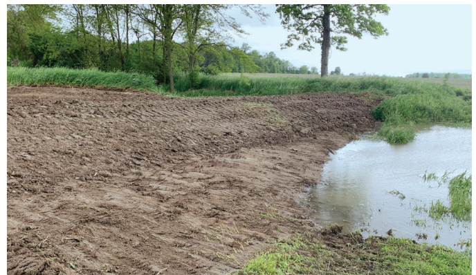
Building temporary dams is one way of containing the material on-site.
