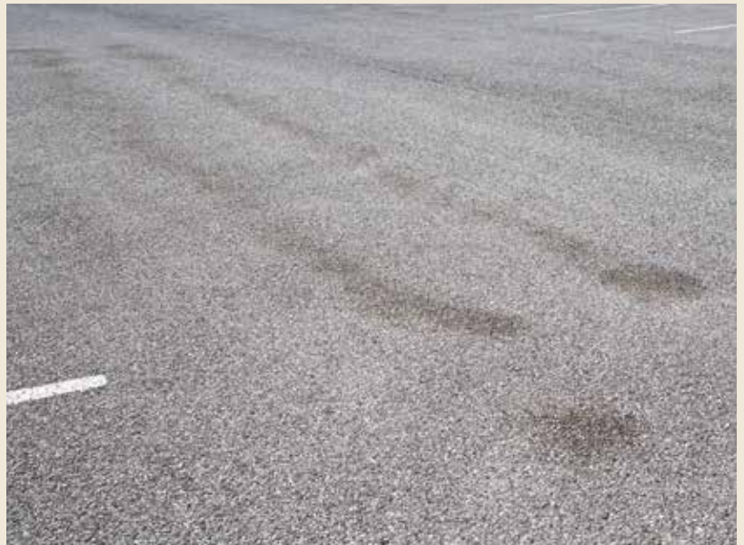
Spraying 5 feet above the pavement is not high enough to deliver an acceptable and uniform pattern.
