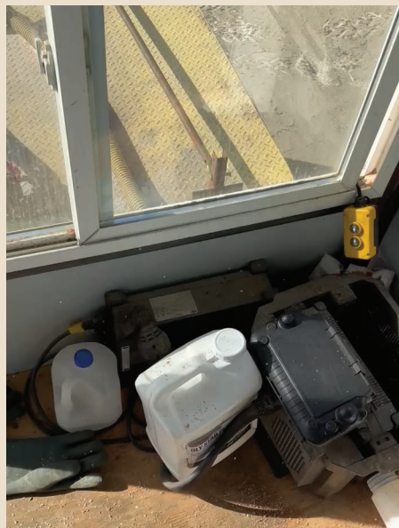
The lift showing the batteries and chargers. Once the day's operations are complete, the drones are brought back into the lift, which brings them down into the trailer.
