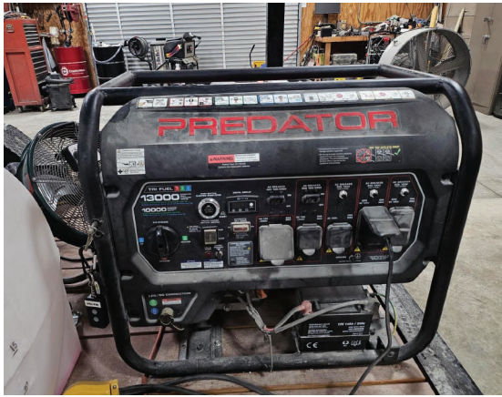
A gas-driven generator generally costs less on the front end, and the lighter weight allows for greater portability.
