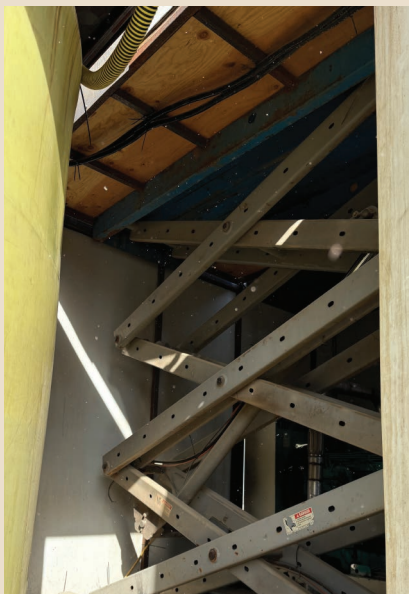
The lift mechanism. The lift is used to bring the batteries and drones to the upper platform.
