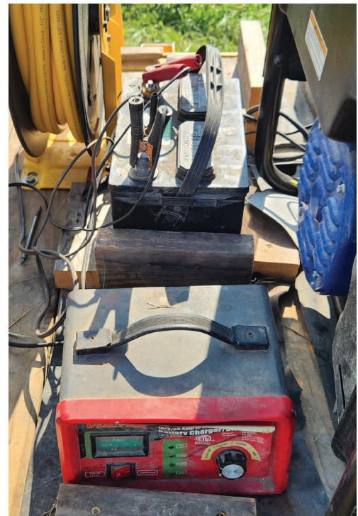
If you use a 12-volt battery to power a pump, you may need a device to convert 120-volt power from the generator to 12 volts to charge the battery.
