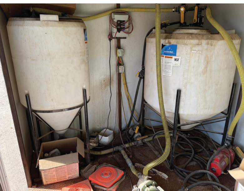
Chemical batch setup inside trailer. Be cautious when utilizing this method to avoid additional exposure risks. Mixing chemicals inside enclosed trailers can cause fumes to irritate the handler. Ensure proper ventilation if your tanks and chemical jugs will be opened inside.
