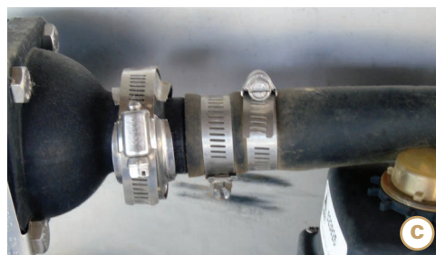
(A) A limitation of standard clamps is that at some point they can be stripped if the screw is tightened too much. (B) These pressure hoses have two standard clamps with the two screws aligned with each other. (C) A better method is to have the screws opposite each other, which allows the weaker area around the screw to be offset by a tight "round-on-round" section of the neighboring clamp.
