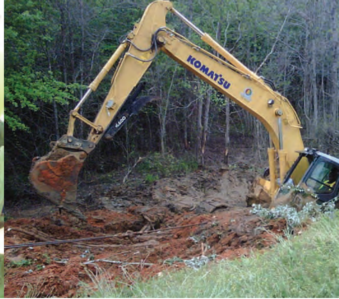
The operators are using two cables to pull this vehicle out of a quagmire.
