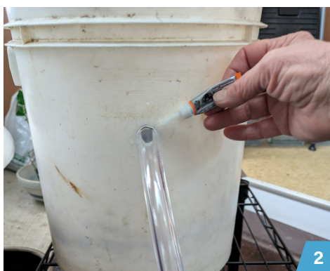
Add glue around the hole to prevent leaking
