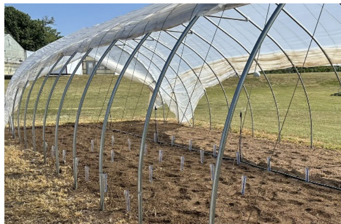
Figure 26. Multiple rain gauges are placed in the tunnel to assess irrigation uniformity.
