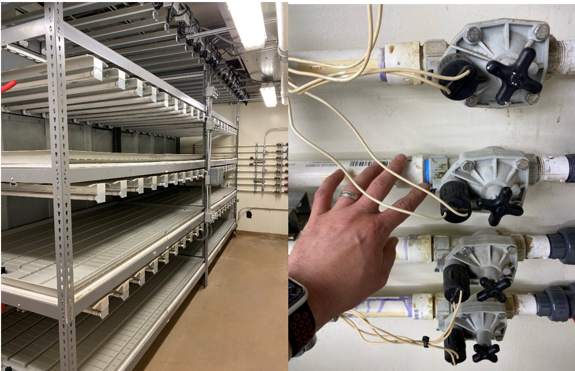
Figure 3. Side View of Rack Systems
