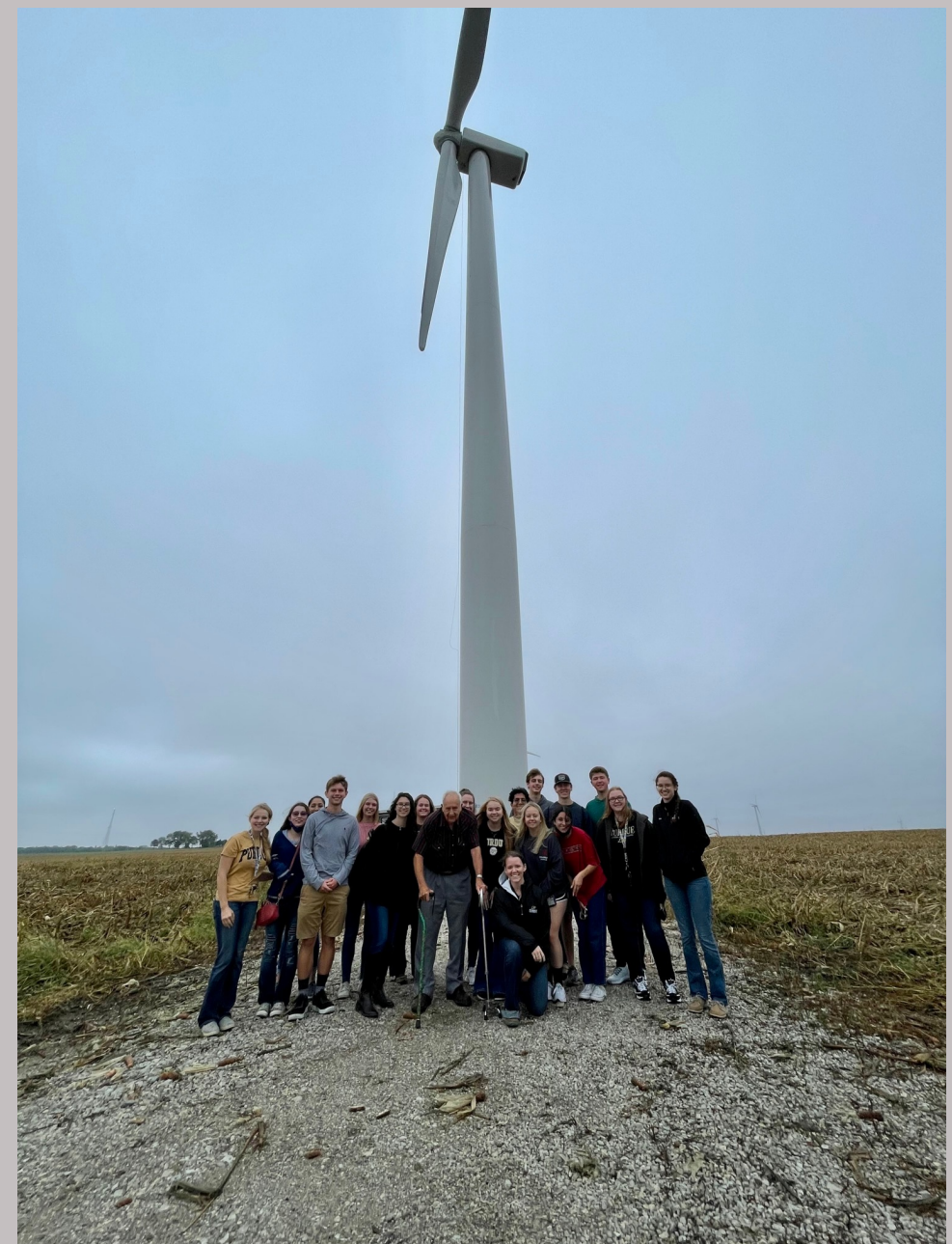
Benton County Wind Farm
