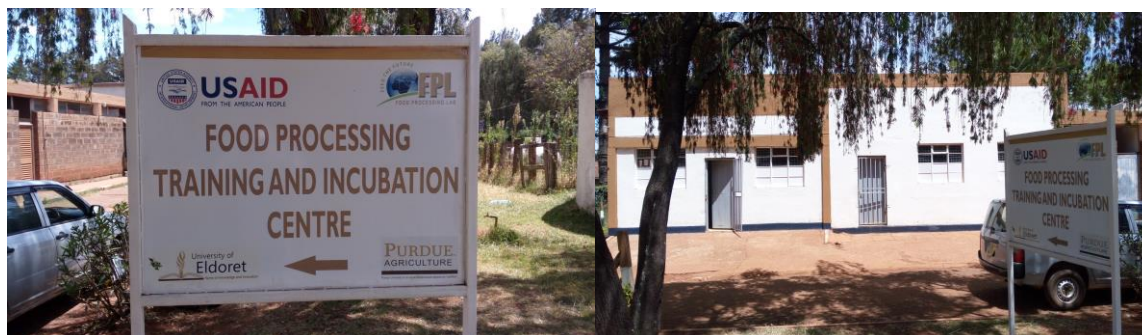
Figure 8. Food Processing Training and Incubation Center (FPTIC) at Univ. of Eldoret in Eldoret, Kenya. Facility equipped with destoner, dehuller, milling machine, decorticator, extruder, dryers, baking ovens, refrigerator, and electric cooker.
