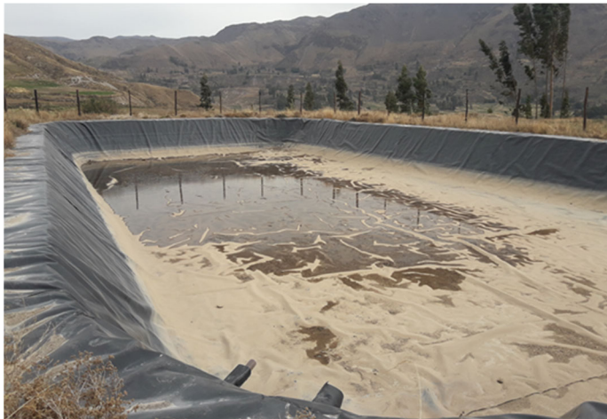
Reservoir in Lari at the end of the dry season
