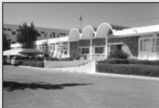
Administration building at Institut des Régions Arides, Tunisia.
