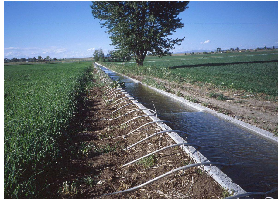
Lined Ditch with Siphon Tubes
